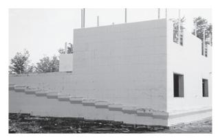
The various form units have cores of 4" (102mm), 6" (152m), 8" (203mm), 10" (254mm) and 12" (305mm), with an overall thickness of  $9\ 1/4"$  (235mm),  $11\ 1/4"$  (286mm),  $13\ 1/4"$  (337mm),  $15\ 1/4"$  (387mm) and  $17\ 1/4"$  (438mm) respectively. The BLE can be used at any elevation on the wall on either side. The form is 32" (813mm) long x  $13\ 1/2"$  (343mm) deep.
